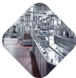
COMMERCIAL DAIRIES & DAIRY PROCESSING PLANTS
